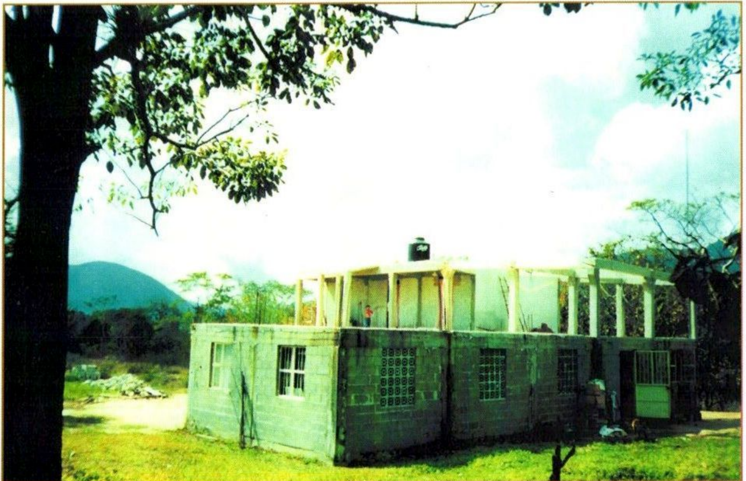
The office, classroom, and dormitory in progress
